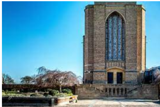
St Mary's University Chapel Waldegrave Road, Strawberry Hill TW1 4SX
